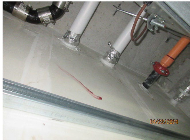
Floor A-49 = Wall pipe penetrations F/S & S/S
