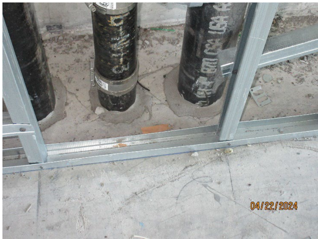
Floor A-55 = Floor pipe penetrations F/S & S/S
