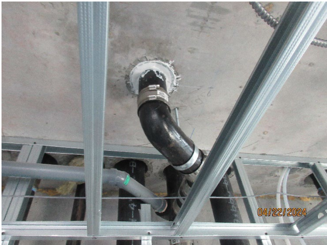
Floor A-55 = Drain pipe penetrations F/S & S/S
