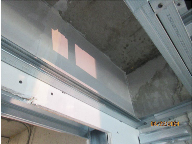
Floor A-56 = Top of Drywall Fire caulked
