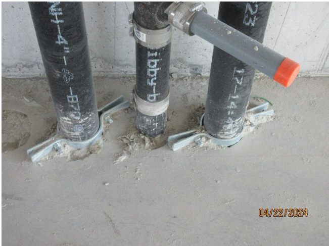
Floor A-58 = Floor pipe penetrations F/S & S/S
