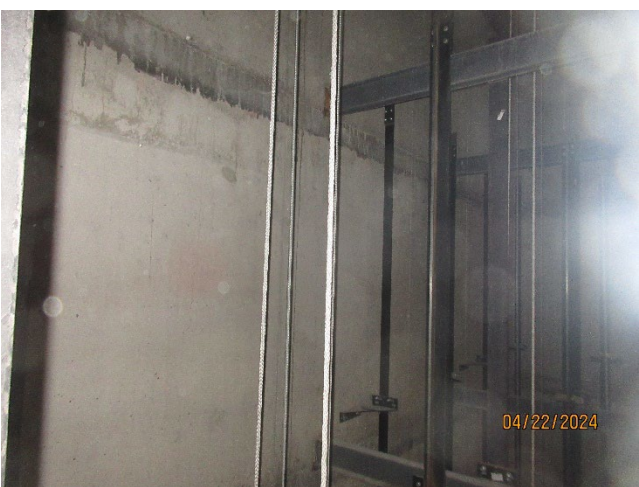
Floor A-57 = Elevator guide rails
